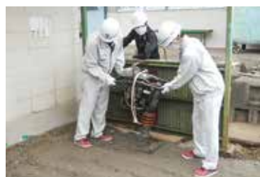
⑫路床締め固め
